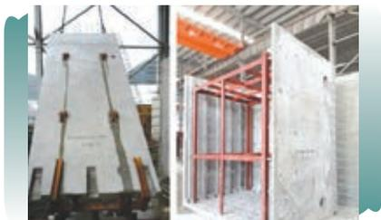
Precast elements construction system is widely adopted in our construction sites. As they are prefabricated in mass volume off-site, the volume of in-site concrete could be substantially reduced, which means the associated pollution generated in the course of concreting can be either reduced or saved. In one of our active construction sites, over 6,500 trees have already been saved through prefabrication adoption.
